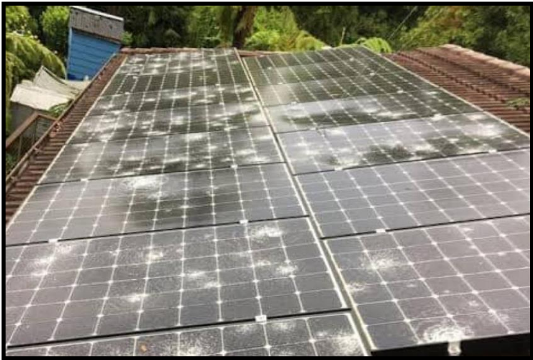
“The damage to property after the hailstorm passed over Canberra was extensive, and smashed many rooftop solar panels” (ABC News, 2020)
